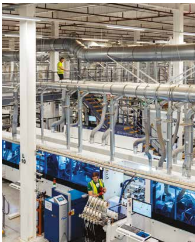
ABOVE Parrott Street factory floor
